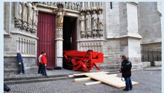
For a better overview the operator can drive the machine with the radio remote control walking alongside the lift.
